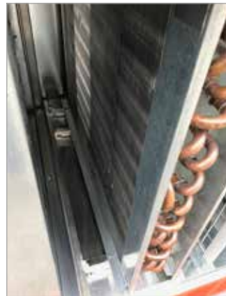
Detail heating section
