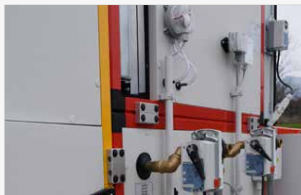
Detail with coil valves, damper actuator, pressure transducer and air quality probe
