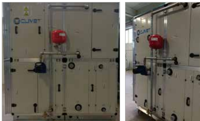
Detail AQX with heat recovery section with fin recuperator
