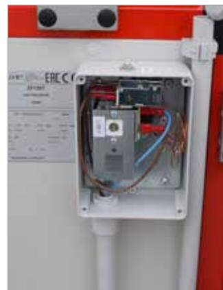
Detail safety thermostat
