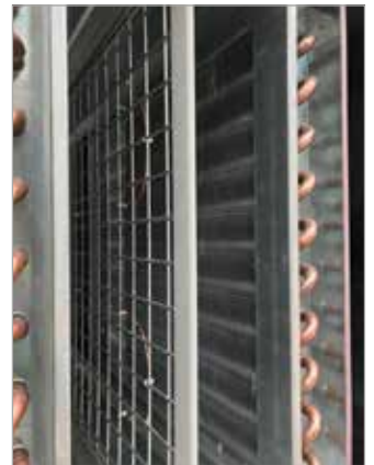
Detail heating section
