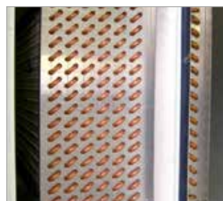
Detail cooling coil
