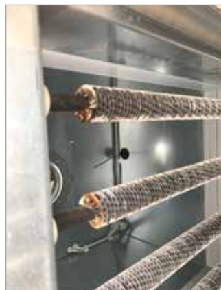
Electric heater elements
