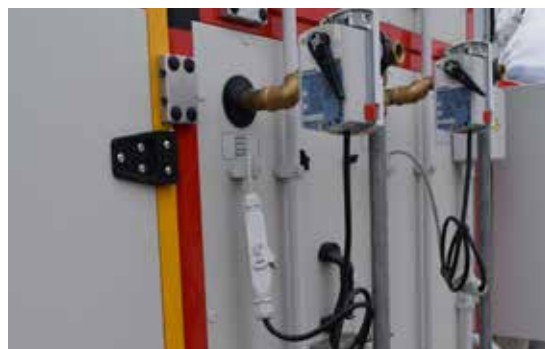
Coil control section
