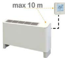
Electrical connection for distances lower than 10m
